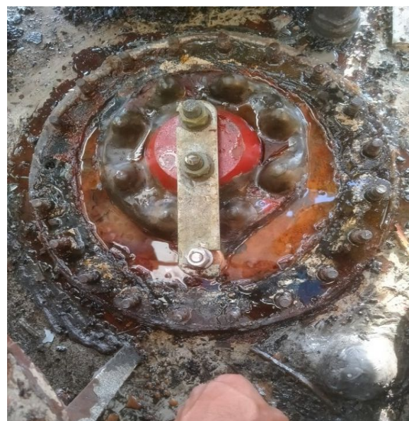
RUSTED CFT CONNECTIONS
