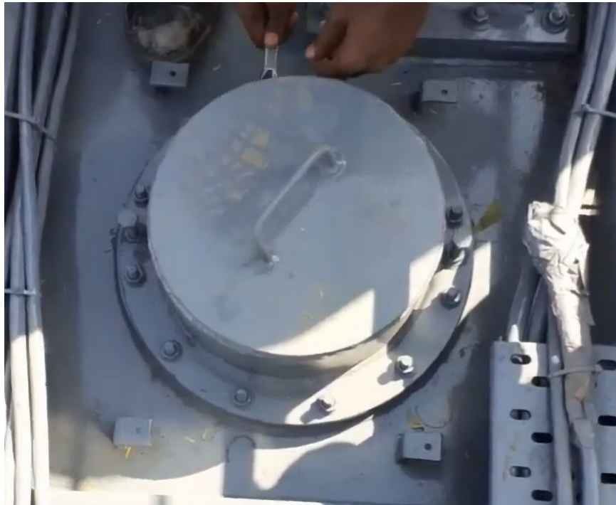
This is how a CFT before Opening Looks like on top of Transformer
