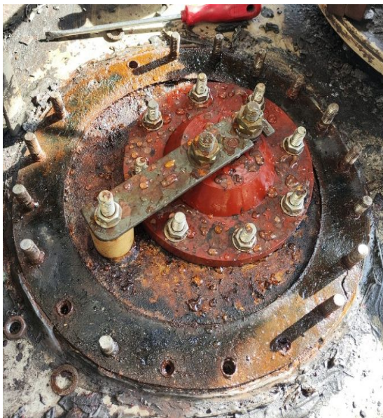
RUSTED CFT CONNECTIONS
